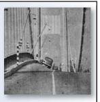
It may cause intense swaying motions and even catastrophic failure in improperly constructed structures including bridges, buildings, and airplanes. The collapse of the Tacoma Narrows Bridge into Puget Sound on November 7, 1940, was due in part to the effects of mechanical resonance.
